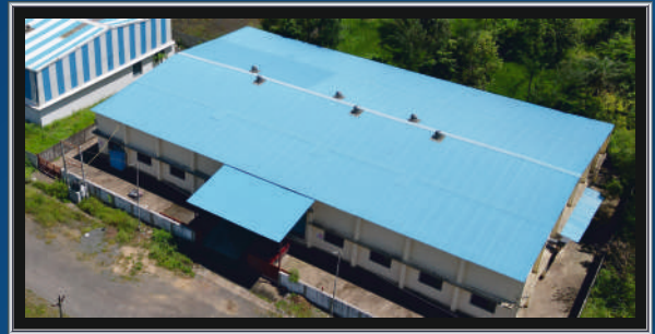
Manufacturing Plant II at Sanjan, Gujarat
